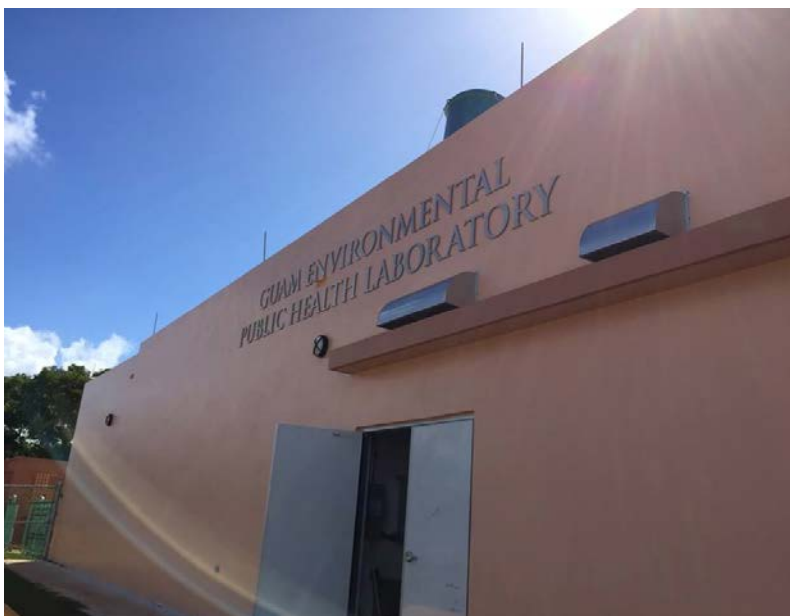
Photo 1. Guam Environmental Public Health Laboratory (GEPHL) building located on W. Santa Monica Ave. in Dededo, Guam. (Source: DEH)
